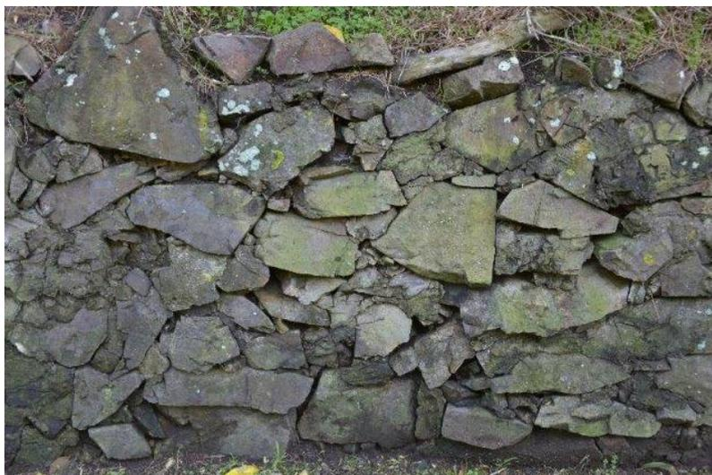
Over the years, stones have dislodged and fallen. Sometimes trees and other vegetation grew within and above the wall, causing damage. The trees were removed a while ago and recently the vegetation was sprayed to assist in the restoration work. The work is expected to be finished later in the year when further funds are available.
