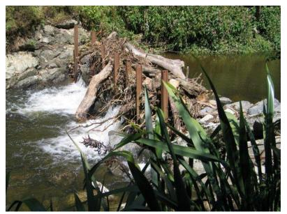
1976 was the year of the great flood in the Kaiwharawhara commercial area down-valley from the Park. Trees, branches and debris carried down by the Kaiwharawhara Stream in spate blocked the tunnel under the oil tanks. The debris trap, as illustrated, was installed. Sam Lister of Capacity organises clearance, prompted by Frances Lee.
